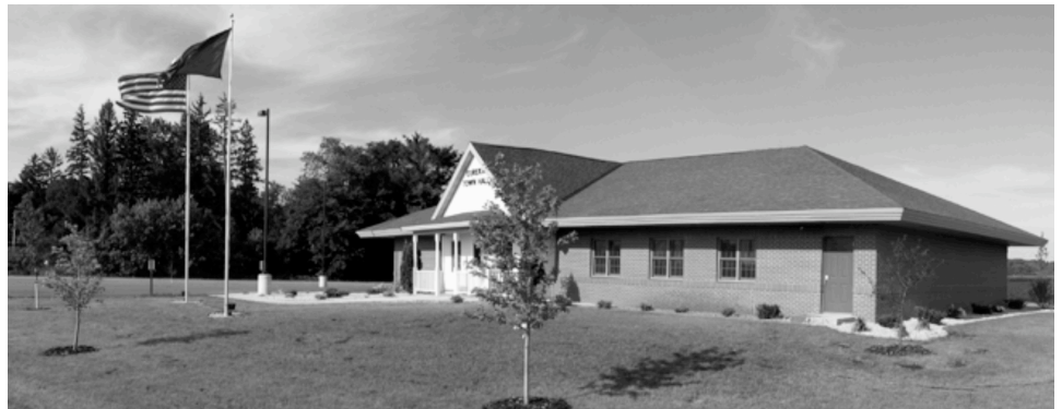
John Strunk, his Strunk Greenhouse employees, and Dan Rogers have installed a landscaping facelift of the Town Hall, drawn up by Dan Cross. Plants, bark, mulch, edging and rock mulch were donated by Cross Nursery, Bachman's, Strunk Greenhouse, and Eureka Sand and Gravel. Existing shrubs were utilized within the landscape.
